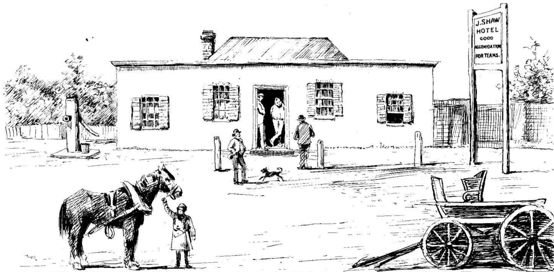
J. SHAW'S HOTEL near Woodbine, KINGSTON ROAD, TORONTO, 1849.
