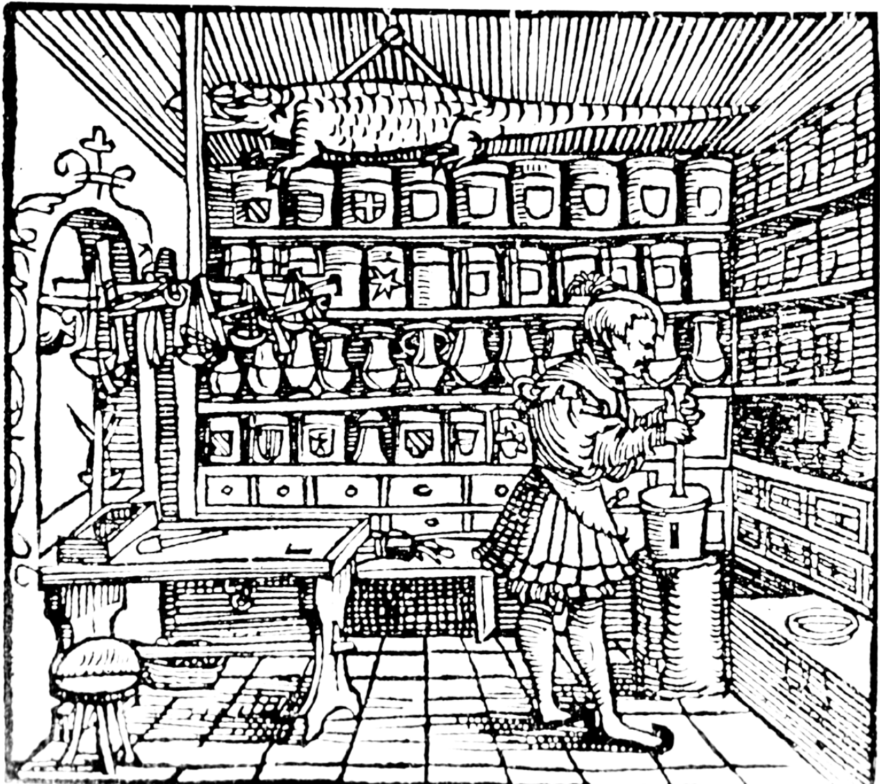
Interior of apothecary shop, 1537
